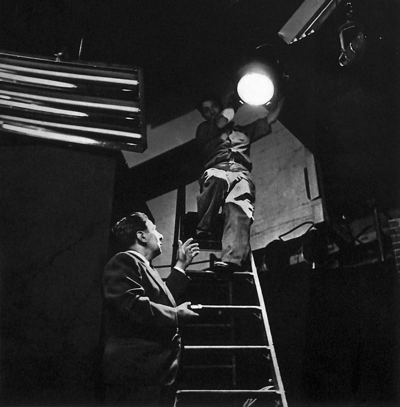
spotlights for accent. Heat and candle-power were cut down by a startling proportion...and a cleaner, better-accented picture came through. Lights are controlled from above, with a catwalk for electricians to work from. Head electrician governs the output of all the lamps in the studio from a central lighting dock, equipped with switch-panel controls.
