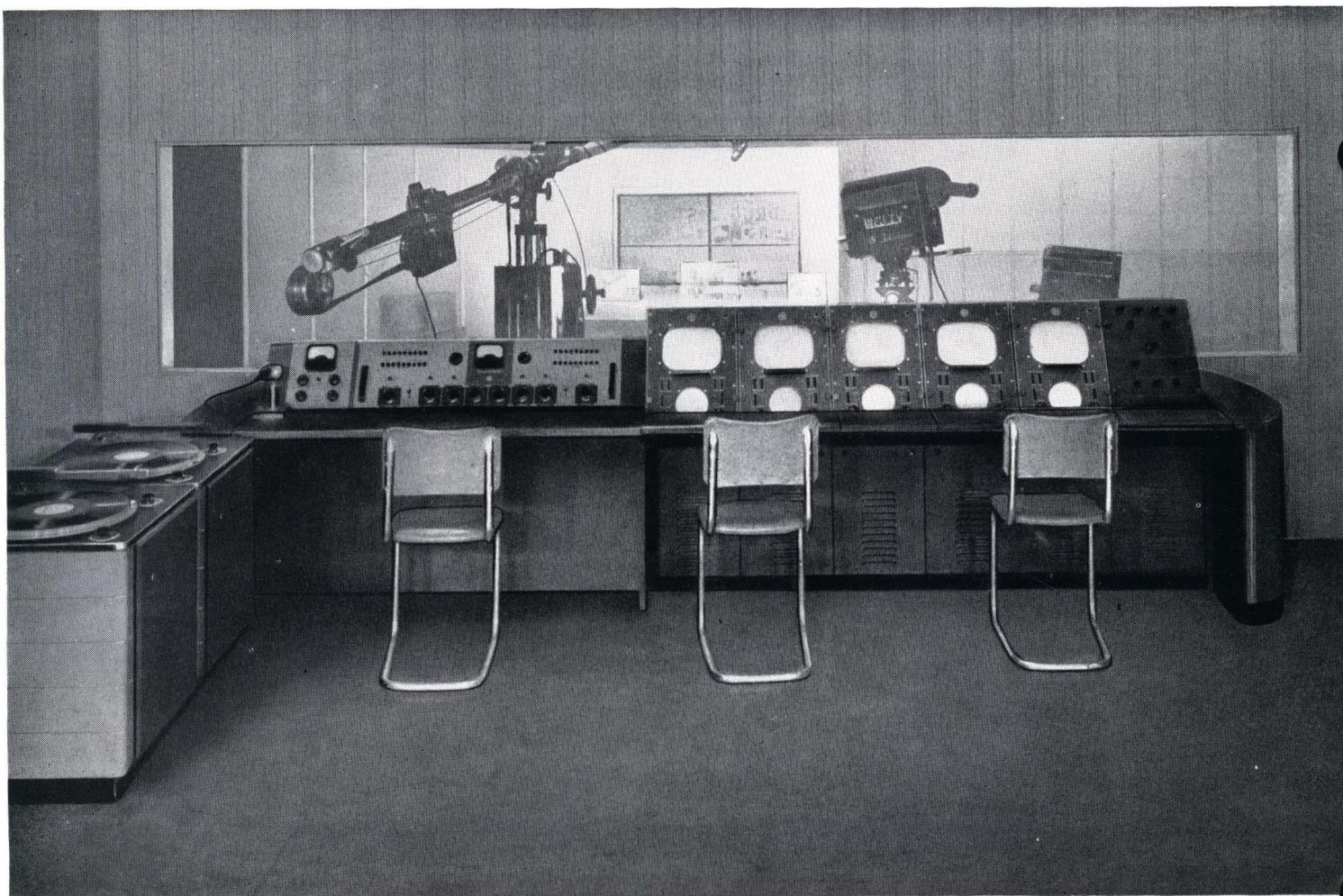
**FIG. 19.** Control Room of the "Standard" or Medium Size Type C Television Station. This station utilizes Studio-type Cameras and control room equipment. In this layout, field-type cameras and auxiliary control units are used for outdoor and remote pickups.
