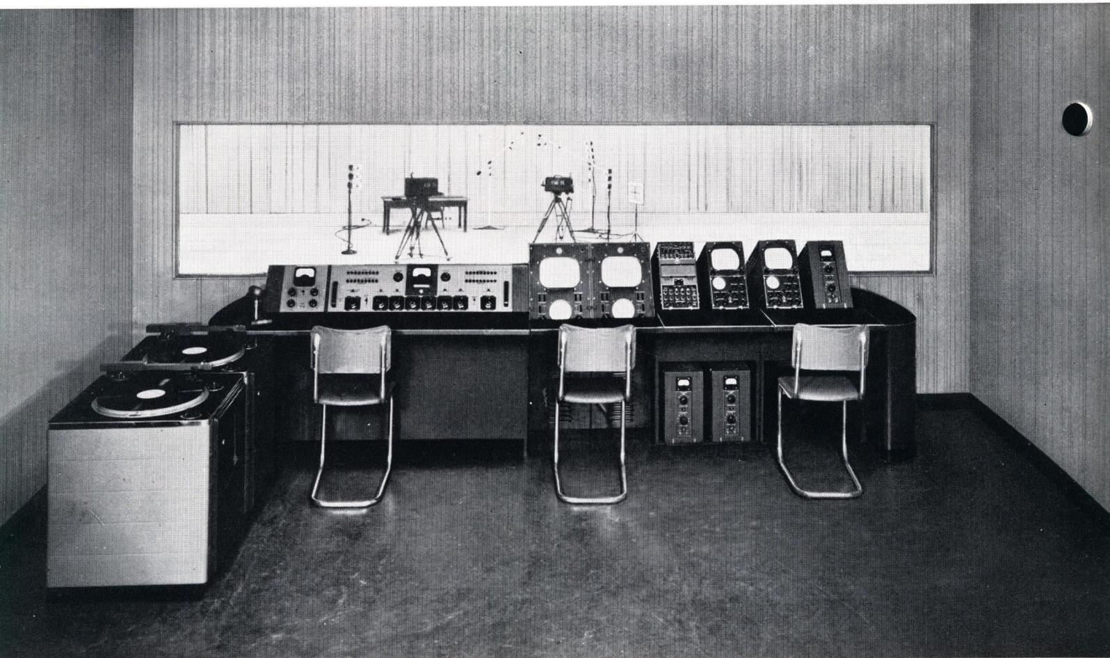
**FIG. 12.** Typical Control Room for the Type A Small Television Station. Two console sections with picture monitors (center) are standard studio control room units. Portable field-type units on the right, when not used for outdoor pickups, are placed in the control room for production of local studio shows. At left are transcription turntables and the audio control console.
