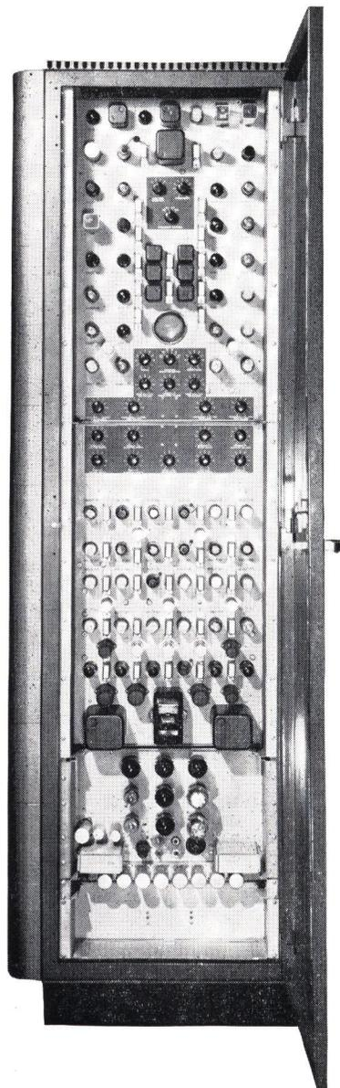
the back of the panels, and are accessible through the rear door. All terminals are in the clear, and components are identified so that circuit testing, when required, is relatively easy.
